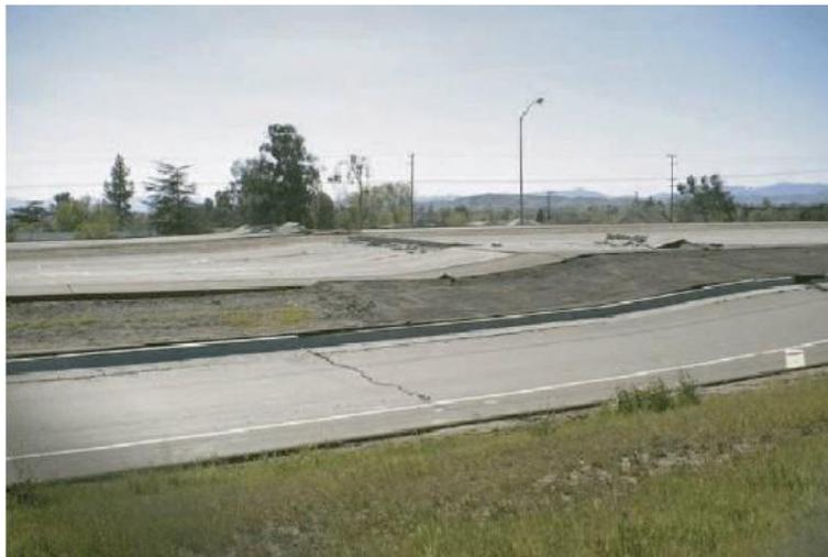
**Figura 1.1** - Recalques em rodovia após o terremoto de San Fernando, em 1971. (Fonte: Researchgate. Disponível em : [https://www.researchgate.net/figure/Settlement-in-a-highway-after-the-San-Fernando-earthquake-in-1971-Courtesy-of-the\\_fig1\\_259466872](https://www.researchgate.net/figure/Settlement-in-a-highway-after-the-San-Fernando-earthquake-in-1971-Courtesy-of-the_fig1_259466872). Acesso em: 15 jul. 2023).
