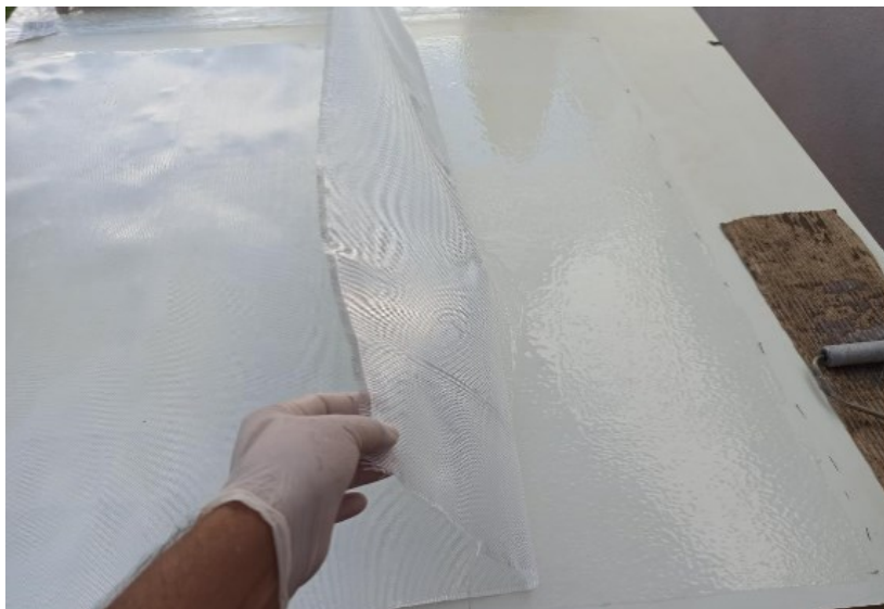
A. 1. Application of a glass-fiber layer [155].
