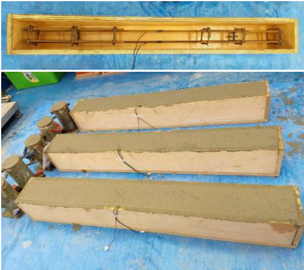
Figure 5-4. Reinforcement positioned at wooden formwork and beams after concrete pouring.
