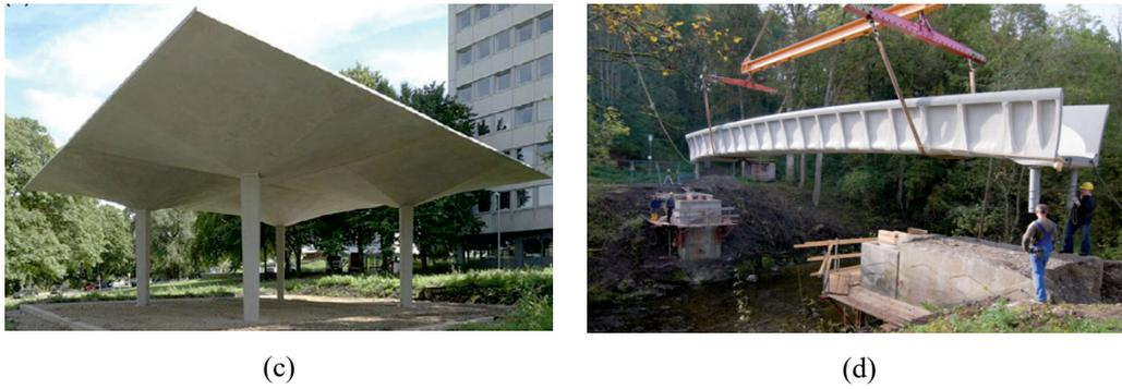
**Figure 2.1 - TRC application examples (a) TRC barrel vault shells as roof elements [47]; (b) Pedestrian bridge Albstadt-Ebingen (solidiam GmbH) [48]; (c) Roof structure of TRC shells at RWTH Aachen [49]; (d) TRC pedestrian bridge [50].**
