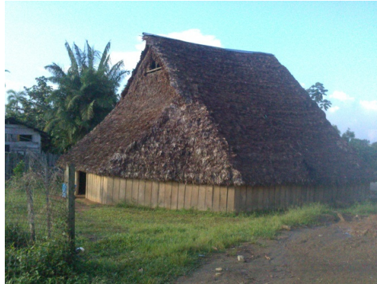
Figure 2.12. Indigenous House, roof built with peach palm leaves.
