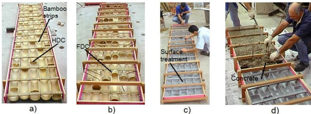
Figure 2.4- (a) formwork of BTDG-HDC (b) formwork of BTDG-FDC (c) epoxy resin treatment [35]
