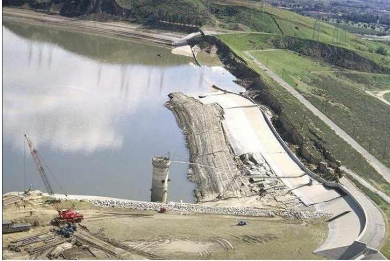
Figura 1.3 Deslizamento na barragem Lower San Fernando, em 1971 (Earthquake Engineering Research Center, University of California, Berkeley, USA).
