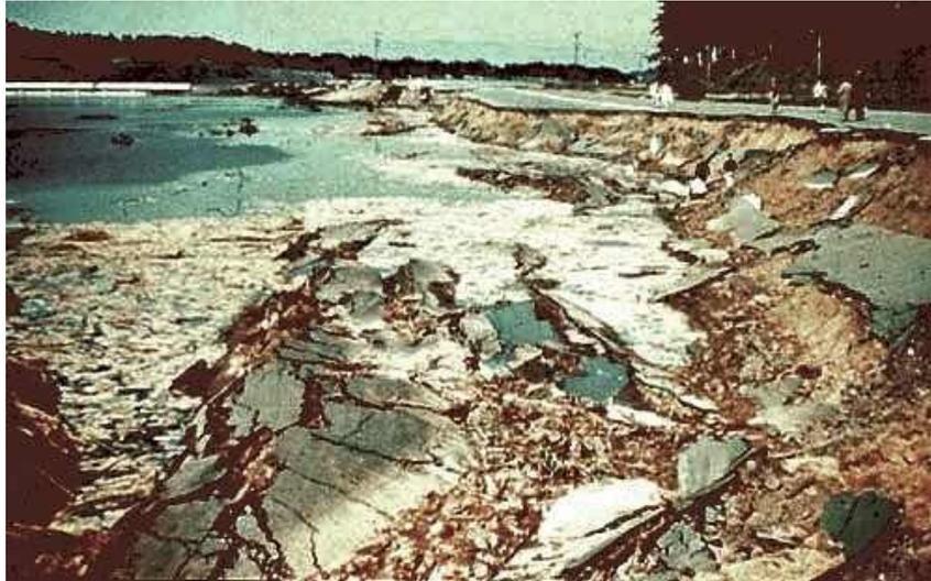
Figura 1.5 Escorregamentos laterais (*lateral spreading*) ao redor do lago Merced, 1957 (Earthquake Engineering Research Center, University of California, Berkeley, USA).
